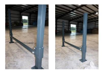
• Once each cross beam has been installed on the posts, proceed to stand up the posts, and have the cross beam at the first set of locks
